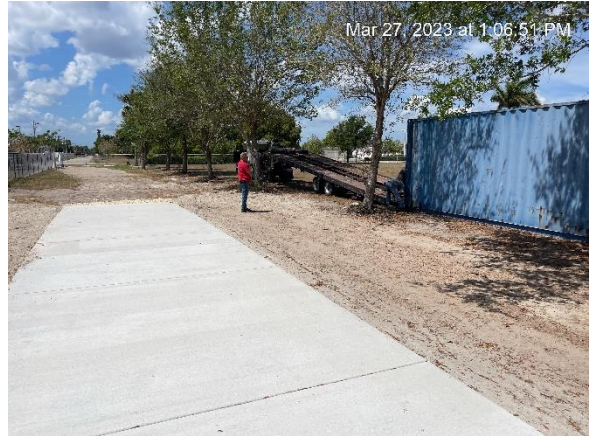
03.27.23 Container Moved to Pad
