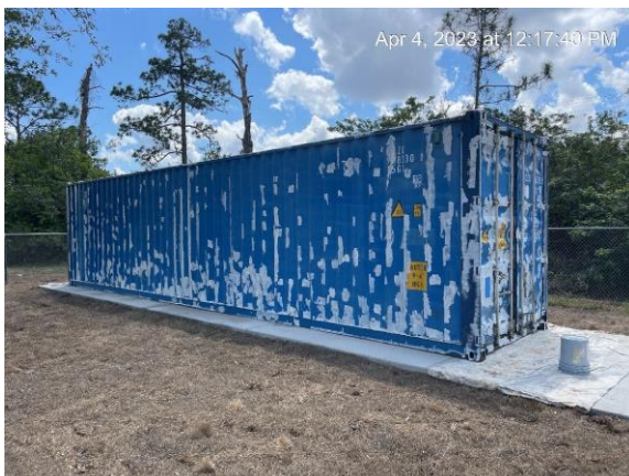
04.04.23 Powered washed for painting
