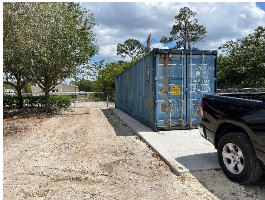
03.27.23 Container with sloping loading pad at doors
