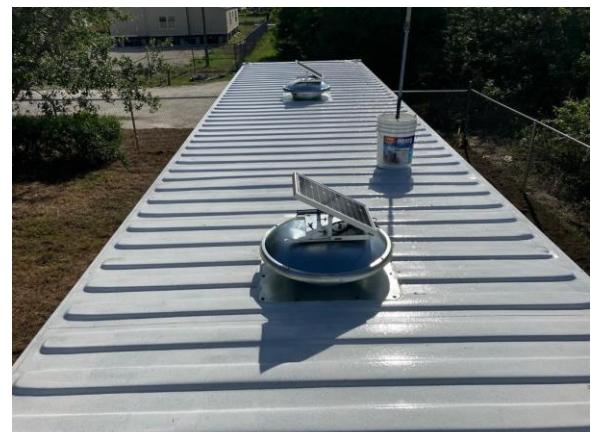
04.05.23 solar powered exhausted fans installed
