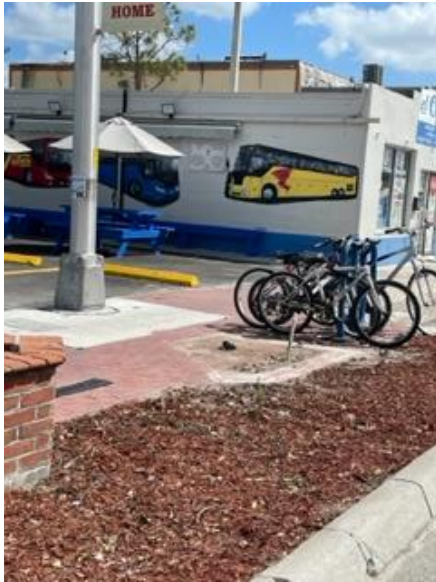
03.27.23 damaged bulbout removed N 3th St
