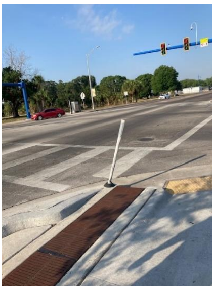
03.13.23 Leaning Pole N 9 th – repaired 3.14.23
