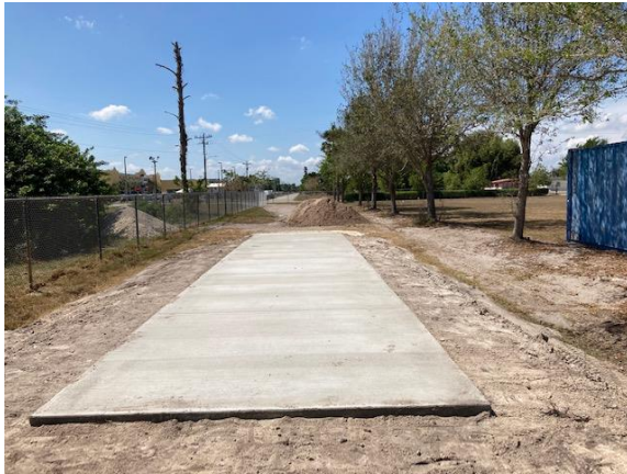
03.13.23 - The Container Pad was poured on 03.11.23
