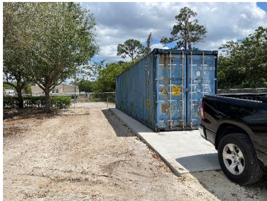
03.27.23 Container with sloping loading pad at doors
