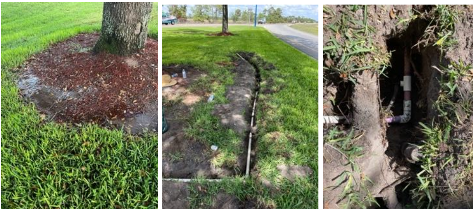
04.06.23 irrigation repairs at the Triangle
