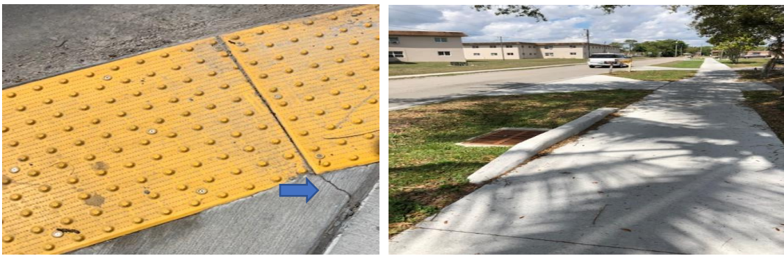
03.17.22 crack under ADA mat NE corner of Eustis/S 5 th and S 5 th St requires a handrail on stem wall
