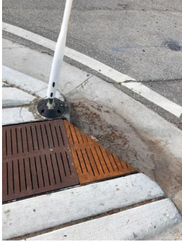
04.07.22 Repaired Grates on W. Main St (3 rd St N pictured)
