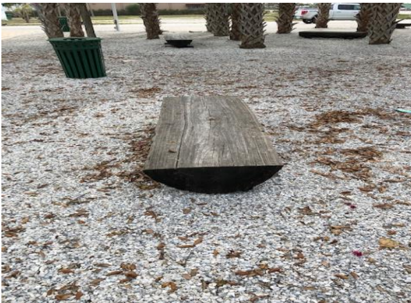
03.11.22 Before – Weathered Appearance of Wooden Benches
