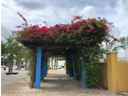
04.01.22 Before - Trimming Bougainvillea on Trellis
