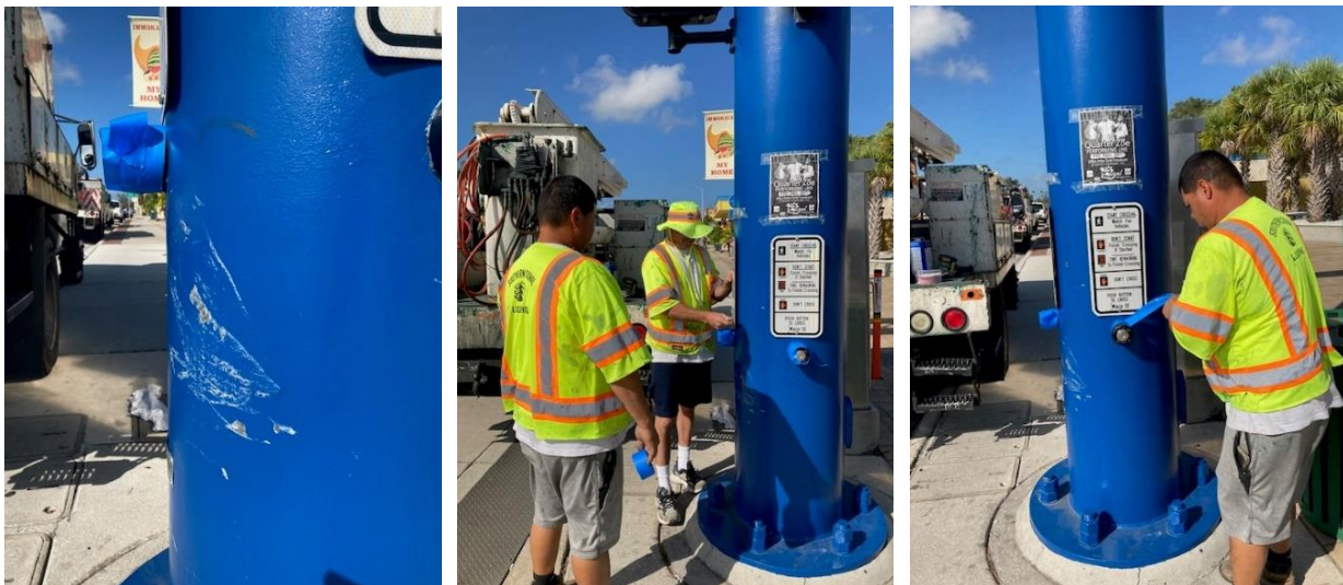
02.09.23 Southern Signal started the work to repaint the vertical pole
