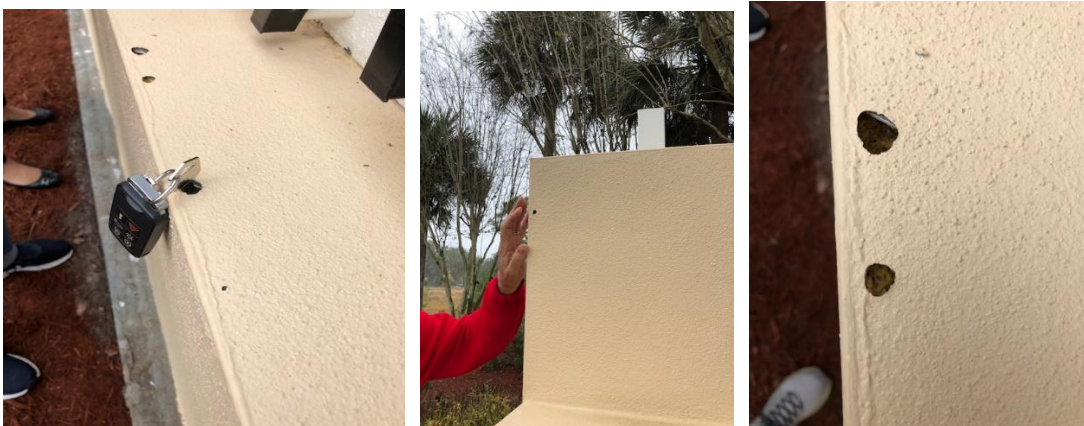
02.07.22 perimeter holes on monument sign
