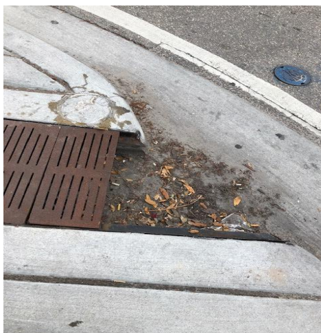
02.07.22 Damaged grate S 2 nd St
