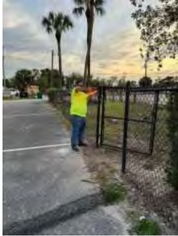
01.16.24 Gate repaired and gate now closes.
