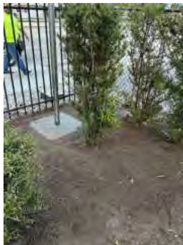
01.16.23 Signage repaired with concrete base
