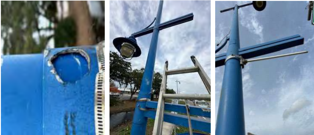
01.16.24 Blue poles aluminum pipes for banner arms repairs
