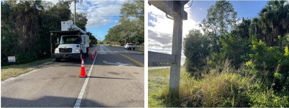
12.18.23 Leaning dead tree at the Panther Crossing Pedestrian Bridge had been cut down.
