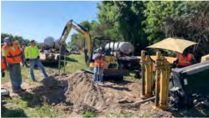
05.04.23 Borning under SR29
