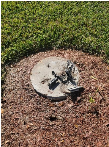
1.10.23 Pole 11 Foundation damaged
