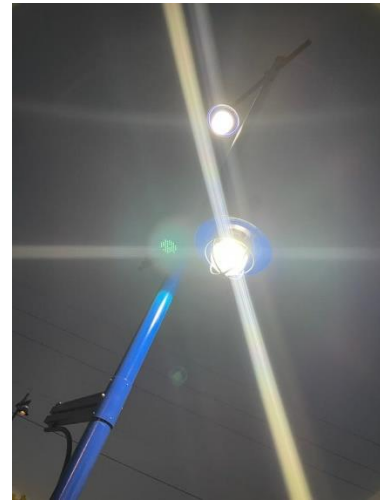
1.10.23 Pole #29 Pedestrian light operating
