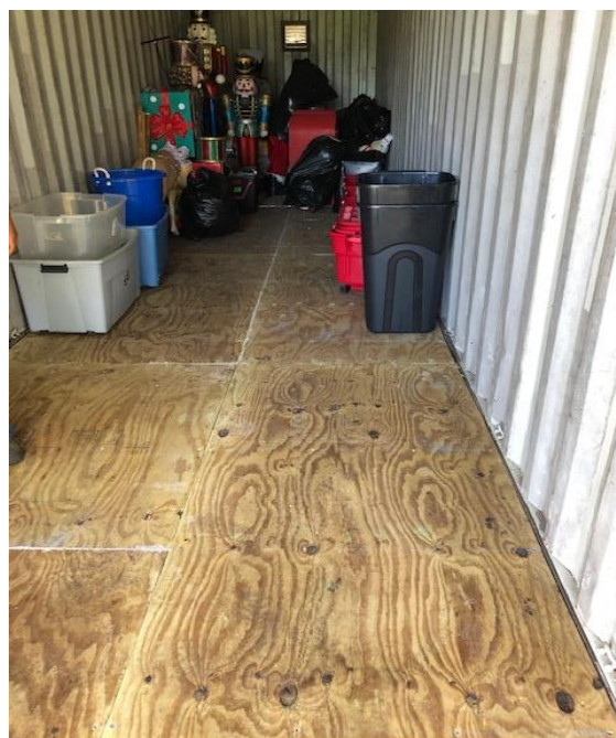
1.10.22 container repairs completed
