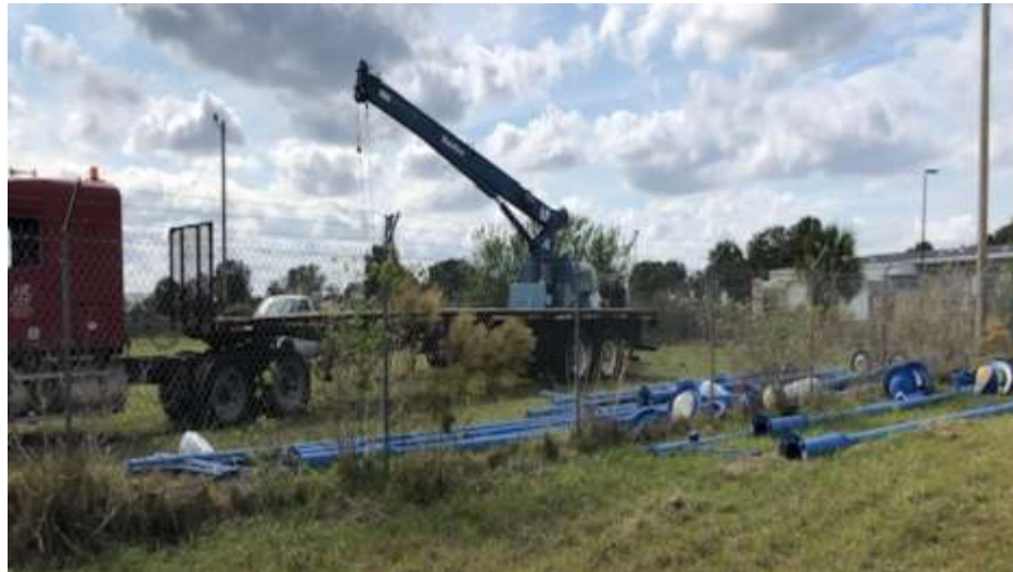
Blue Poles storage area located at Airport 1.11.21.
