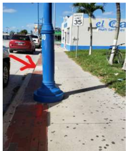
Sidewalk restoration of bricks with removal of blue poles
