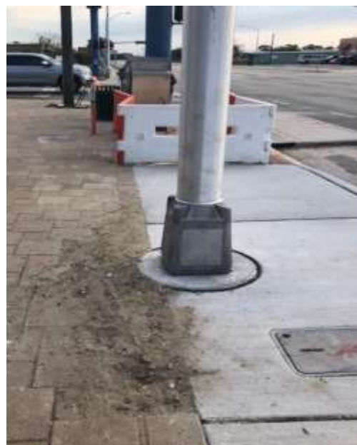
Zocalo new light pole and sidewalk 1.11.21
