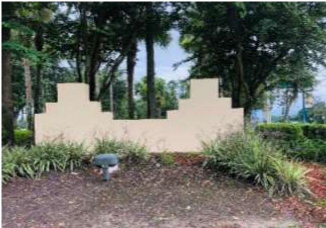
Before plant are installed
