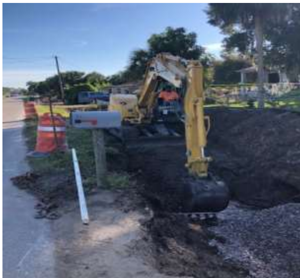
South Side of Carver Photo – December 16, 2020.
