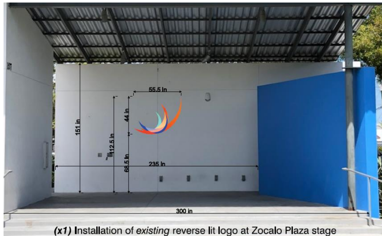
(x1) Installation of existing reverse lit logo at Zocalo Plaza stage
