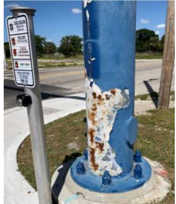
Signal Pole at Main St/9 th St 3.10.21
