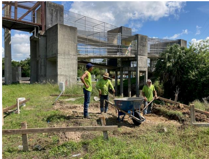
06.14.23 Construction started on the welcome sign.
