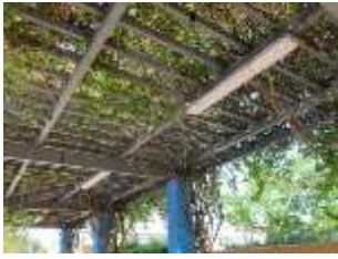
Trellis 3 florescent lights
