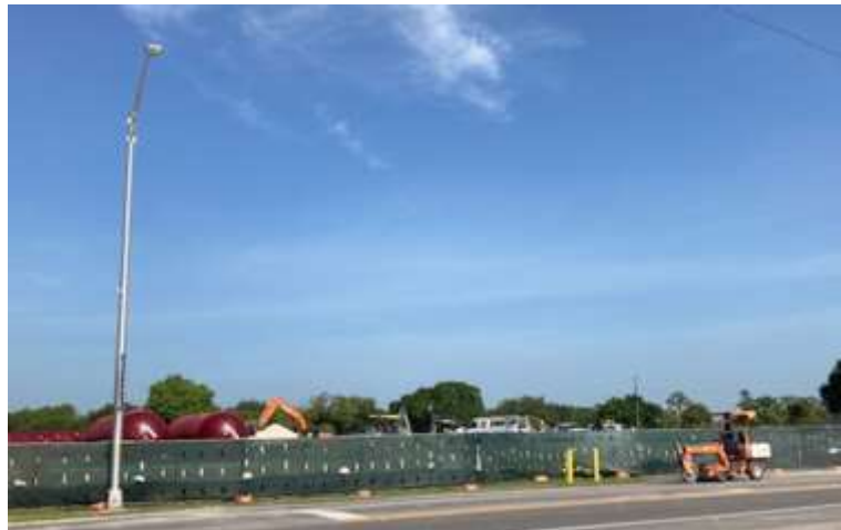
06.13.22 7/Evening preparation for placement of underground tanks and street sweeper
