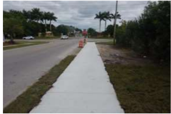
South Side Carver St near Immokalee Rd. 3.9.21
