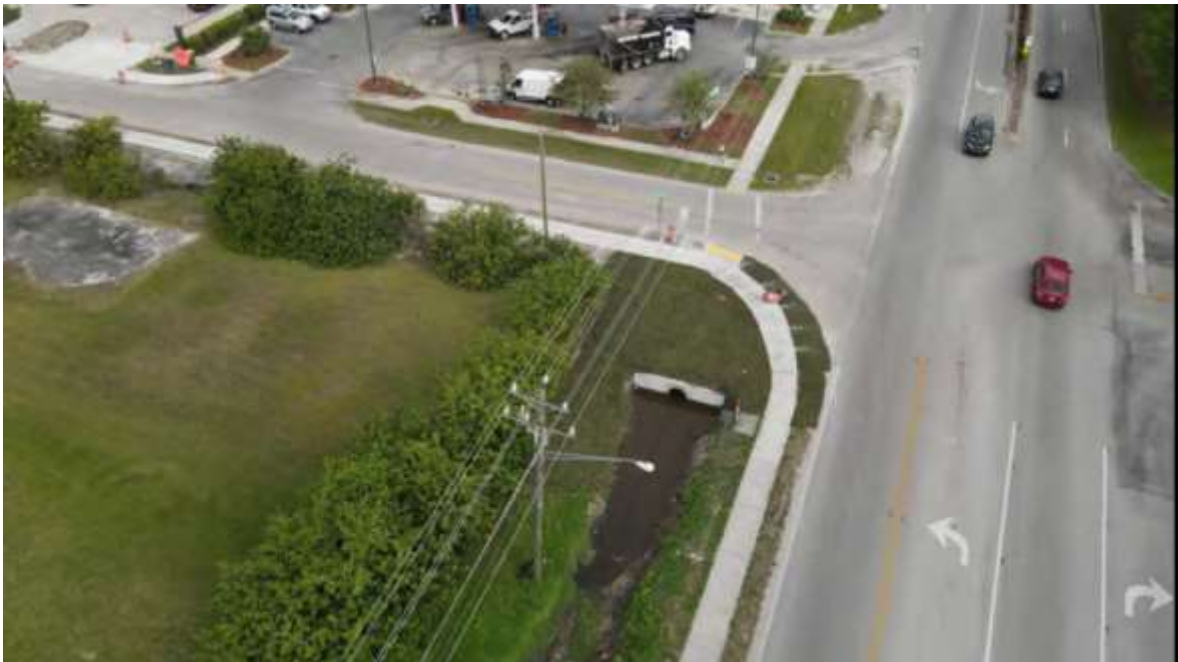
Headwall installed at Carver St and Immokalee Rd. 3.3.21
