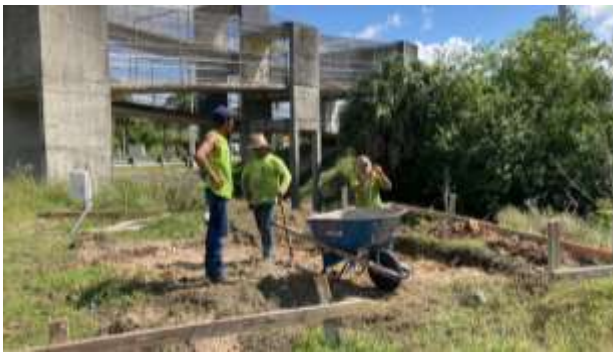
06.14.23 Starting construction of monument sign
