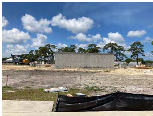
05.01.24 TIGER Project Bus Transfer Station
