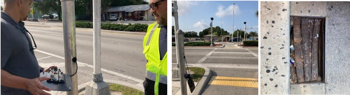
05.13.24 Webber was contacted to repair the signal indicator on 630 W. Main Crosswalk & the storm drain at 208 W Main St.
