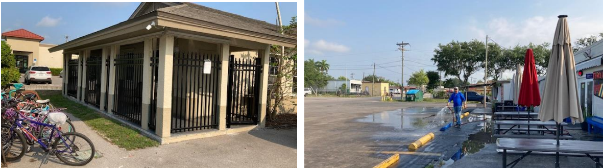
05.13.24 Friendship House installed new alumium black fencing
