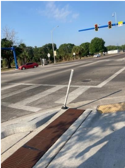
05.08.23 Knocked down delineator S 9 th – reported on 5.8.23, repaired 5.10.23
