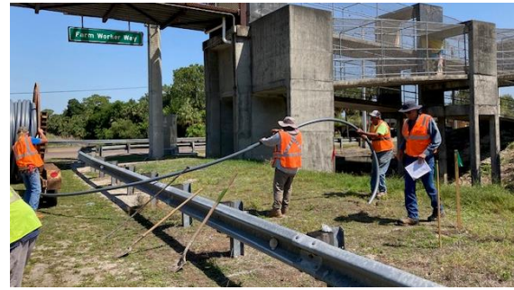
05.04.23 Bore successfully reached the east side of SR 29 and then crossing back under SR29 with pipe to the west side of SR 29
