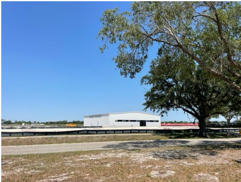
05.04.23 Construction of new Hanger
