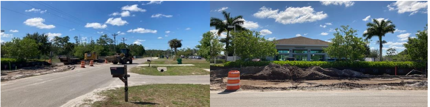
05.08.23 Area 1 - East Delaware Avenue Progress Photos
