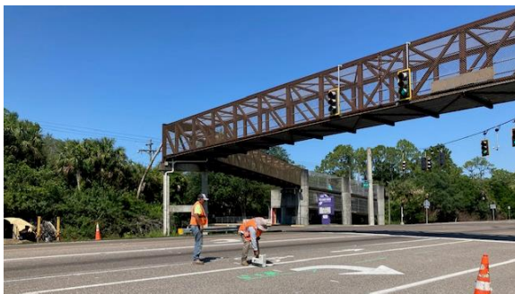
05.04.23 Tracking the bore 3' below the roadway across SR 29
