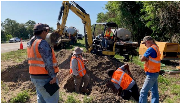
05.04.23 The Preparation to start boring under SR29 to bring water to the signage site
