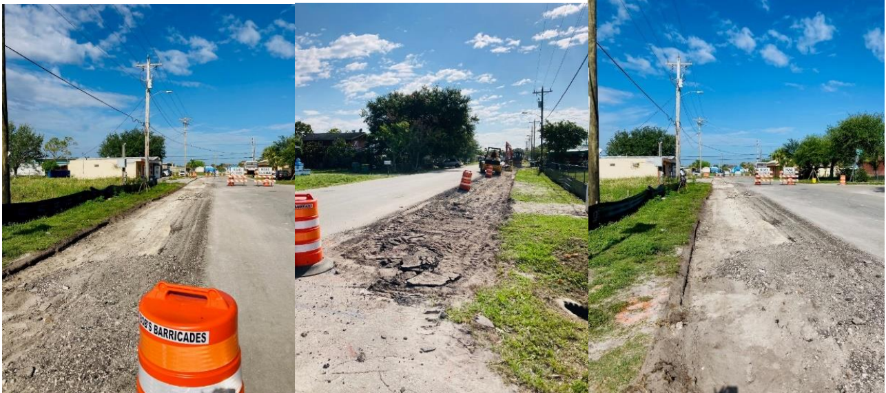
04.26.23 Area 1 - East Delaware Avenue Progress Photos
