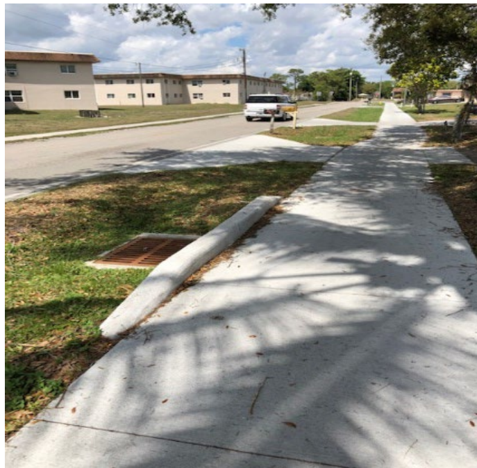
03.17.22 S 5 th St - Post Final Completion a handrail and footer are recommended
