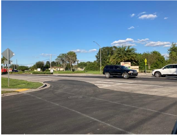
11.01.23 Paving side streets to S 1 st Street
