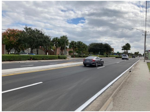
11.02.23 S 1 st Street newly paved
