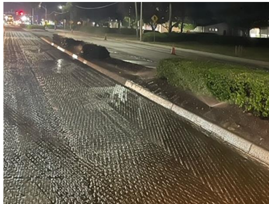
10.31.23 milling the old pavement to resurface.
