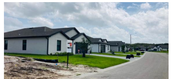
Construction on Arthur Street in Arrowhead Reserve Community.
