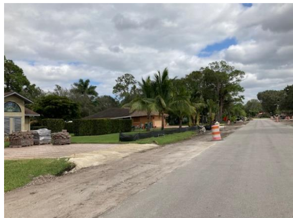
11.02.23 N 11 th Street Sidewalks
