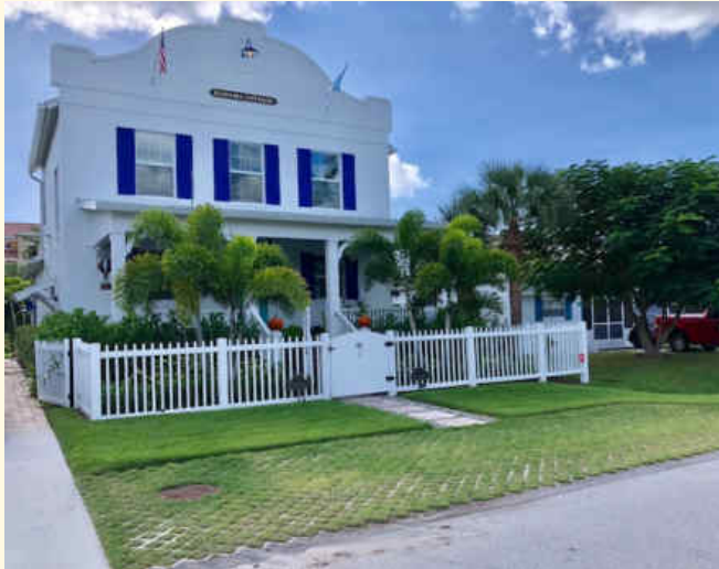
Turf block, shown in the right-of-way area immediately bordering the street in the photo above, has been used in certain developments in the Bayshore neighborhood to allow for use of right-of-way space for parking. This option should be evaluated as part of the right-of-way design considerations in the stormwater master plan update.
