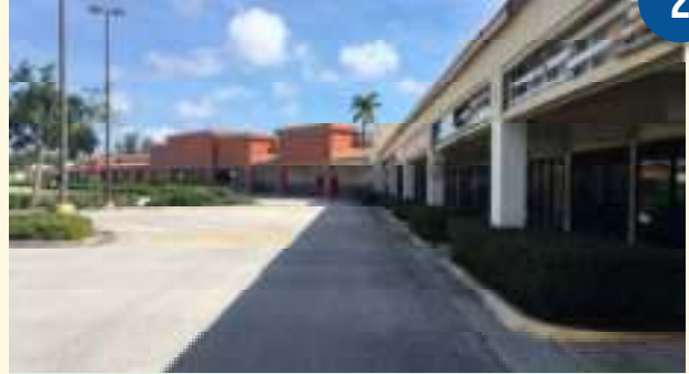
Courthouse Shadows redevelopment
