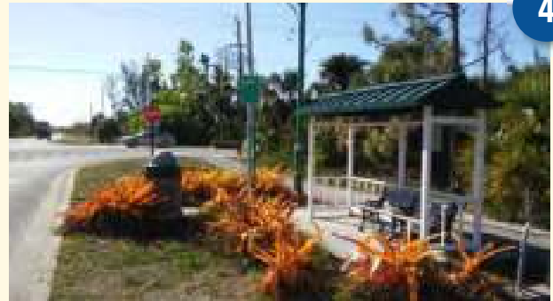
Bus shelter at Bayshore Drive and Thomasson Drive
