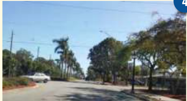
Bayshore Drive commercial corridor redevelopment (including Halde- man Creek Entertainment District near Creek)
