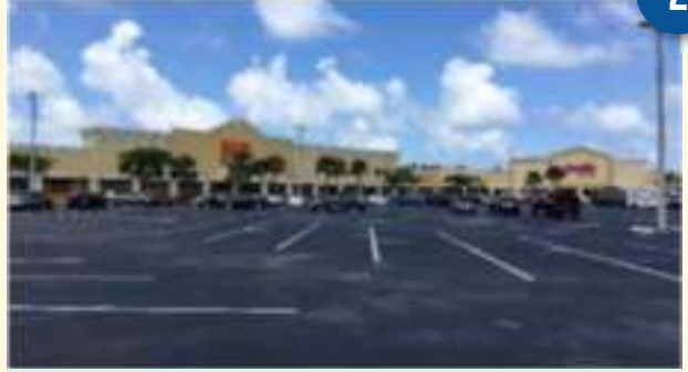
Mall commercial—Gulfgate Plaza
