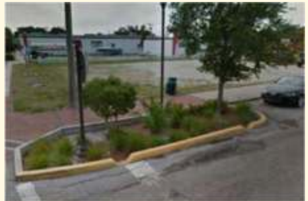
Vegetated infiltration area in roadway bulb-out in Palmetto, FL at 10 th Ave W and 5 th St W (Source: Google Maps, https://www.google.com/maps/@27.5151522,-82.575633,3a,60y,118.29h,75.57t/data=!3m6!1e1!3m4!1slahqGivzSzLDetQ43h5HQg!2e0!7i13312!8i6656 )
