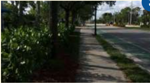
Bayshore Drive with sidewalks and bike lanes
