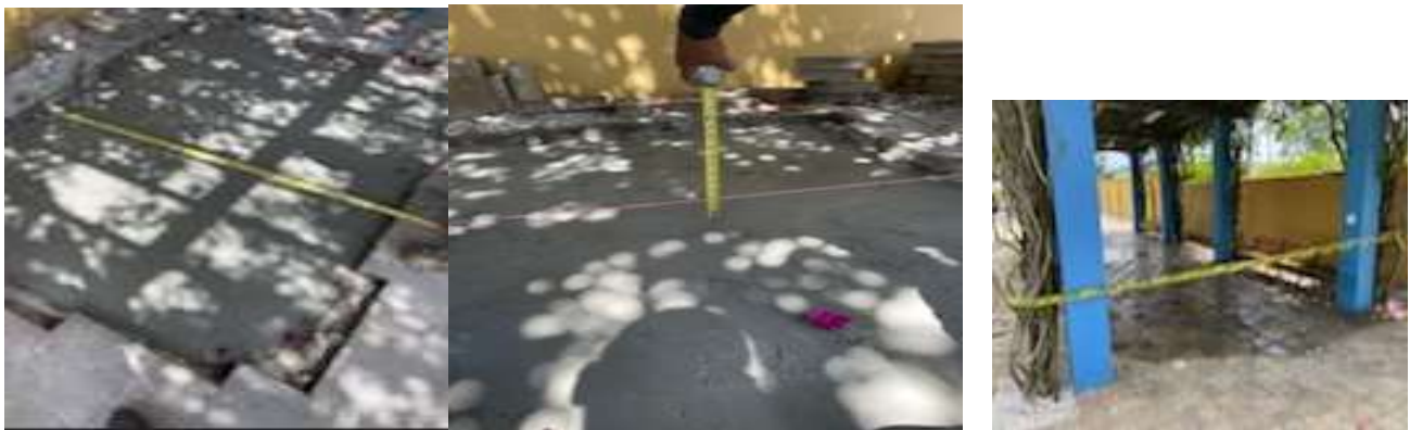
8.20.22 Memorial bench installation – paver removal, poured concrete pads & reinstallation of pavers
