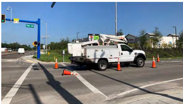
07.10.23 Southern Signal crews working on Main/9 th poles.
