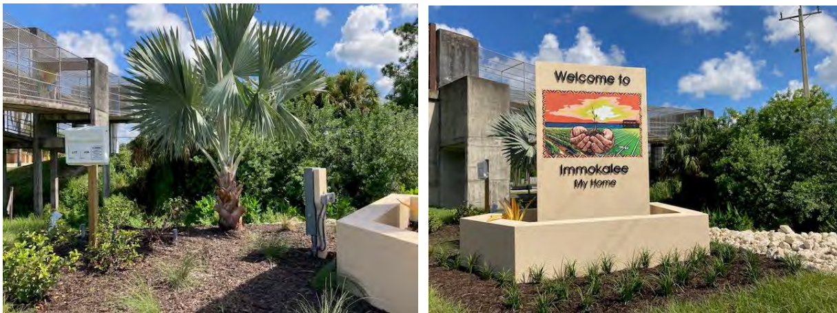
09.08.23 Installation of tree at welcome sign
