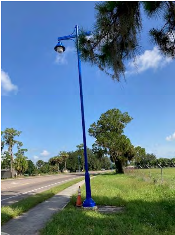
07.10.23 Pole #20 installation complete
