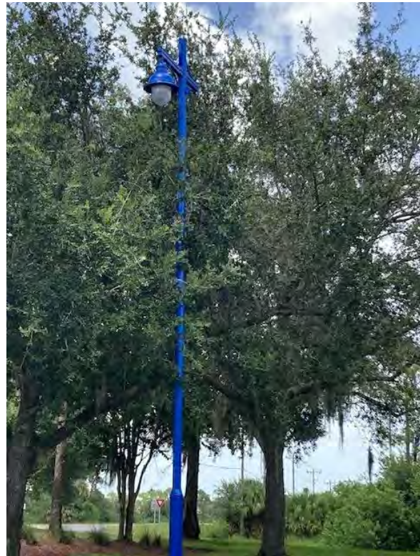
08.22.23 Pole #7 at the Triangle installation complete
