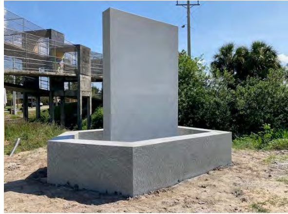
07.06.23 Stucco completed and ready for paint on 07.07.23
