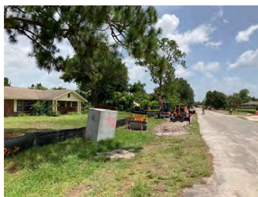
08.22.23 TIGER construction at Monroe and Lee
