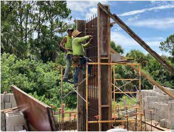
06.23.23 Vector Contracting constructing the sign
