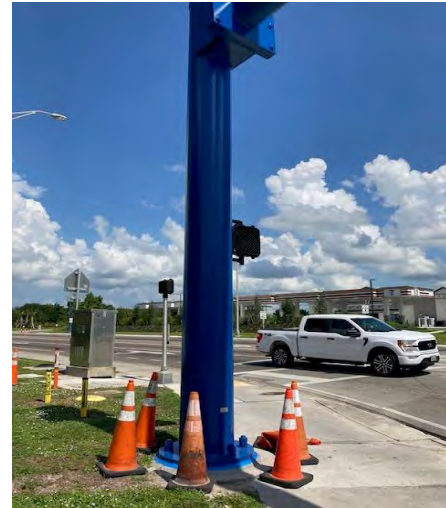
07.06.23 SW Pole Upright Painted at Main/9 th
