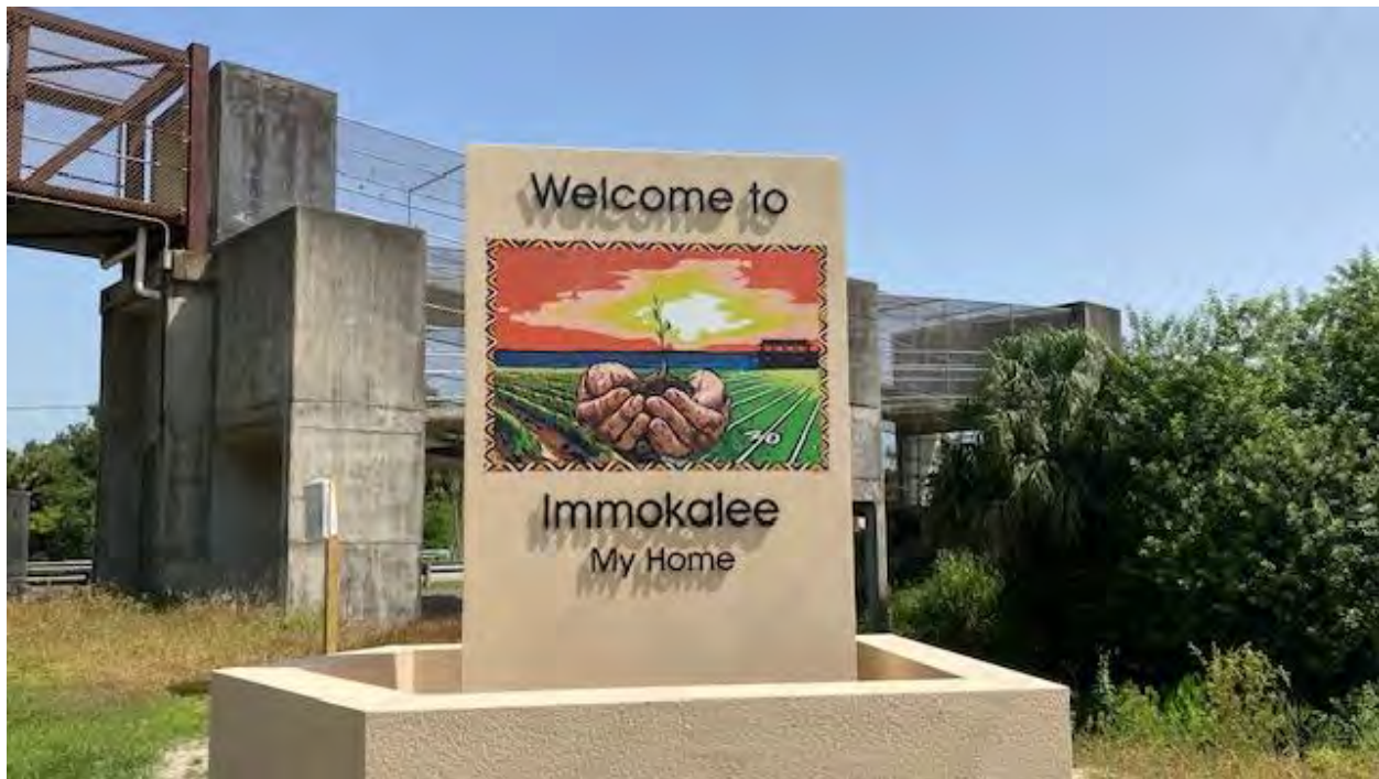
07.25.23 Panther Crossing Welcome Sign under construction.
