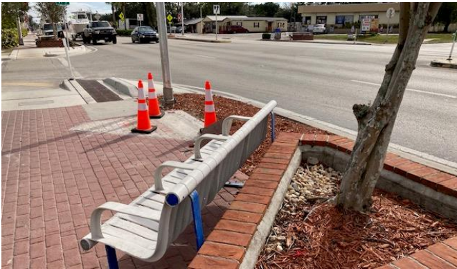
01.07.25 A&M had removed crash debris and PVC pipe, cut rebar, poured concrete to smooth the surface
