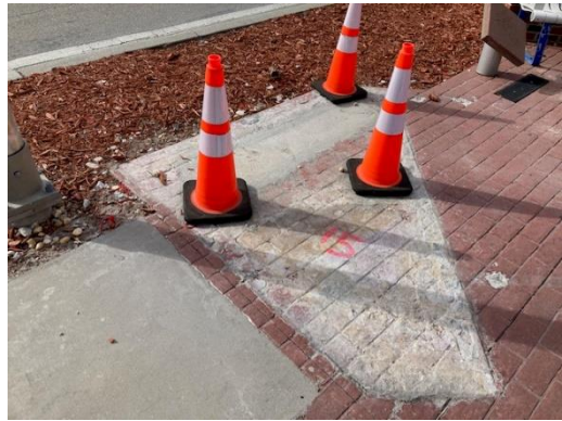
01.07.25 A&M had removed crash debris and PVC pipe, cut rebar, poured concrete to smooth the surface
