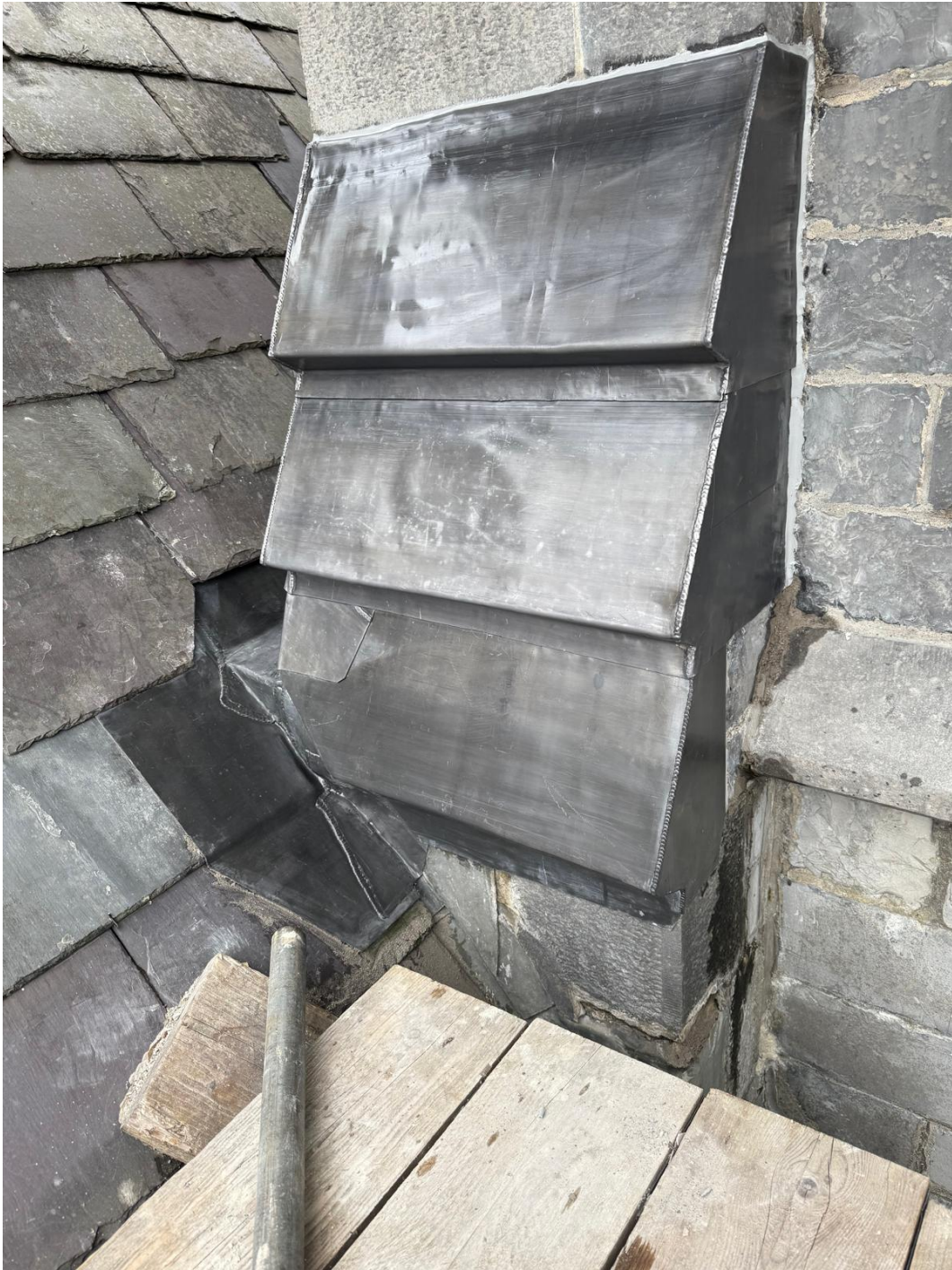
Lead cladding on top of buttress
