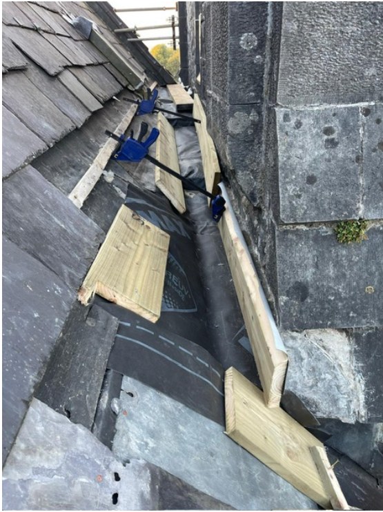
Lead valley: Works in progress
