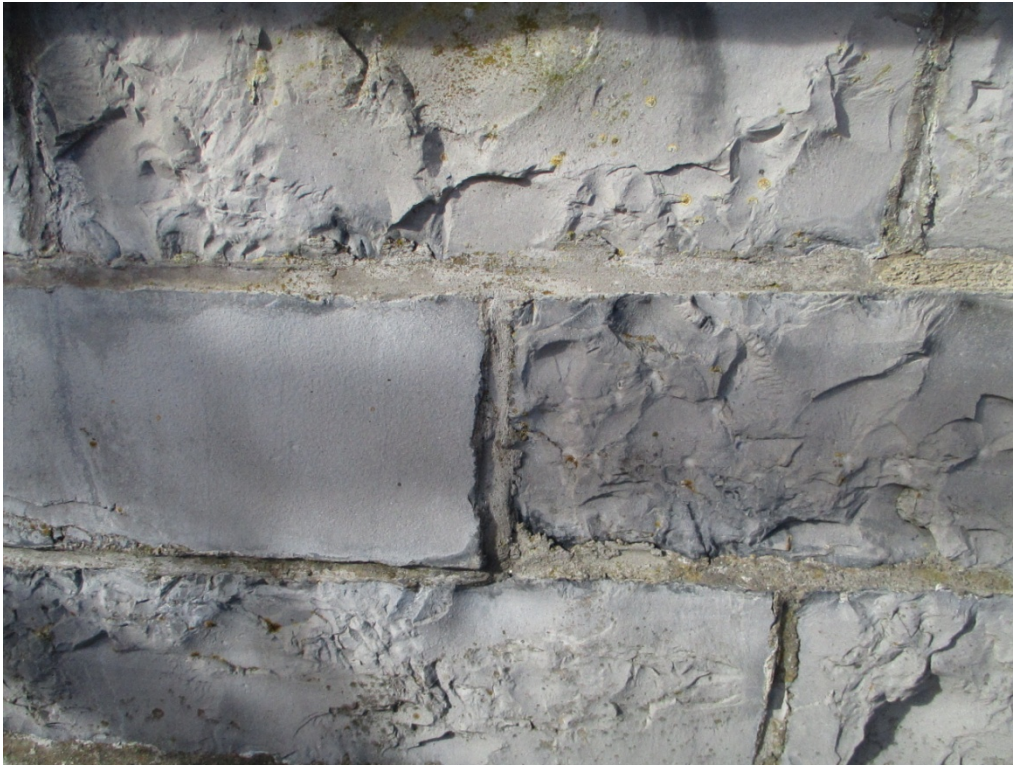
Detail of re-pointing of masonry on tower
