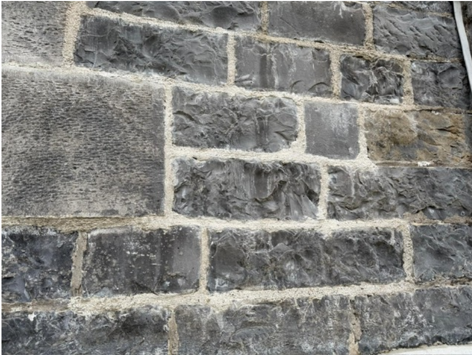
Re-pointed panel of stonework on tower
