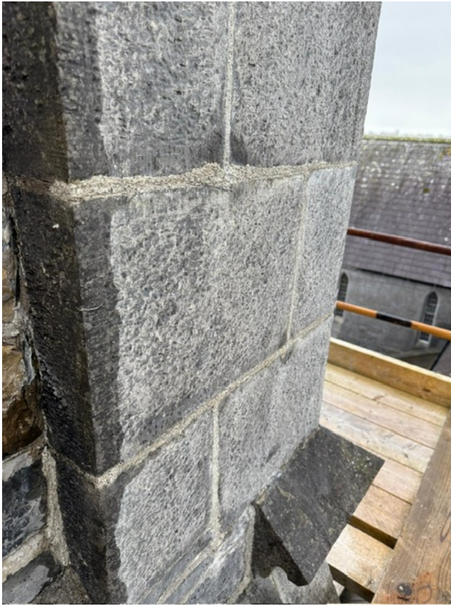
Detailed of re-pointing of masonry on corner of tower
