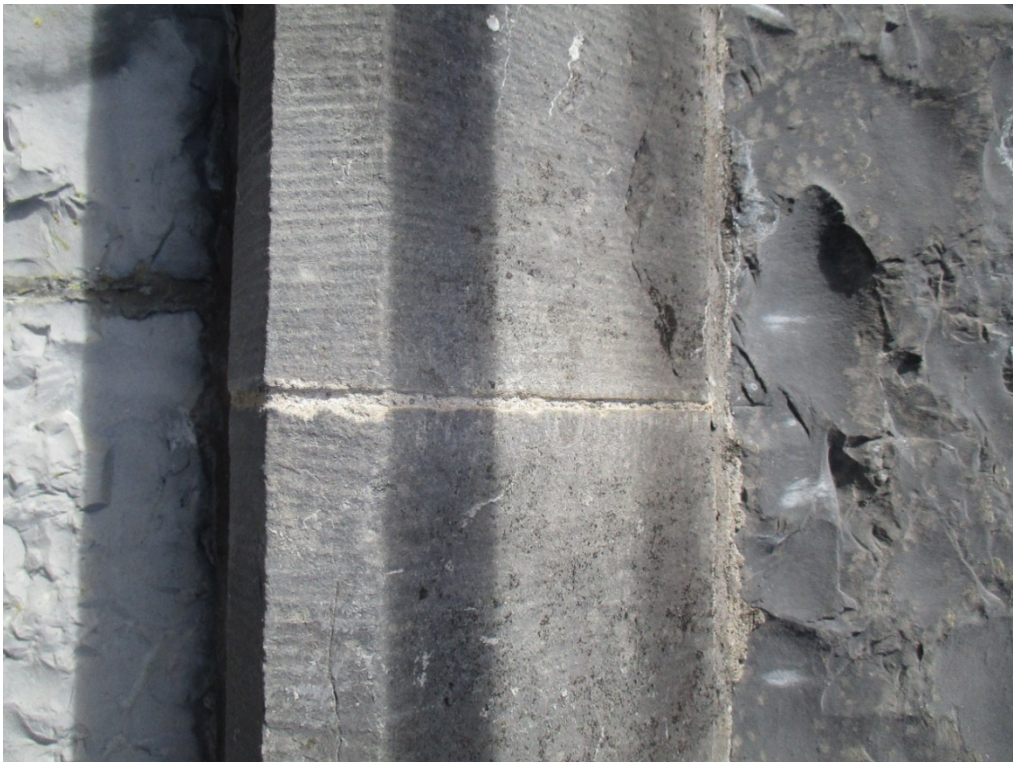
Picture of re-pointing of masonry on tower
