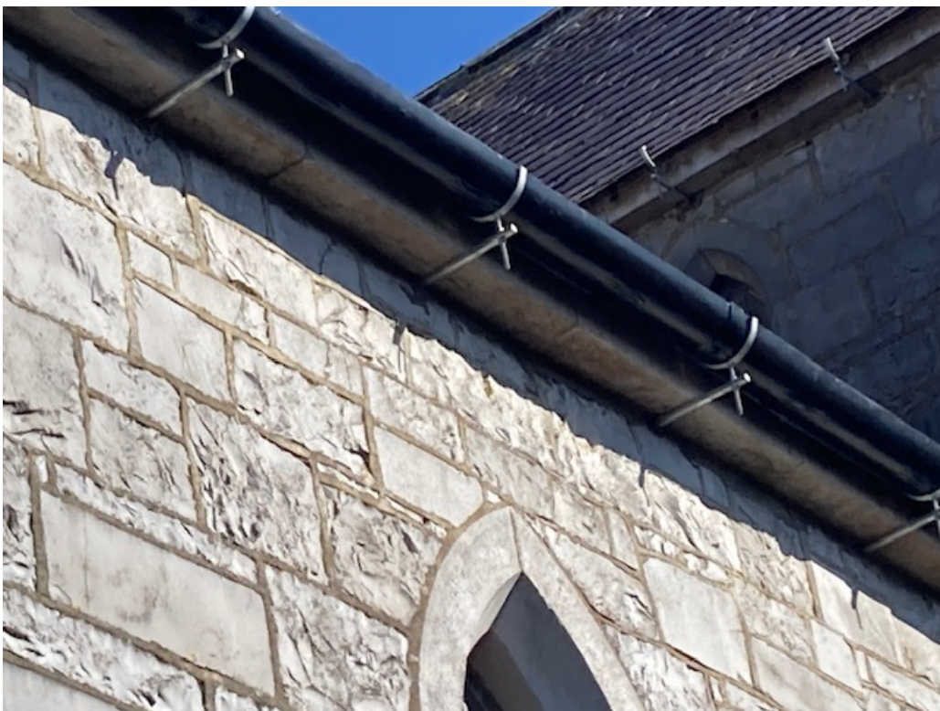
Detail of completed gutter and replacement brackets
