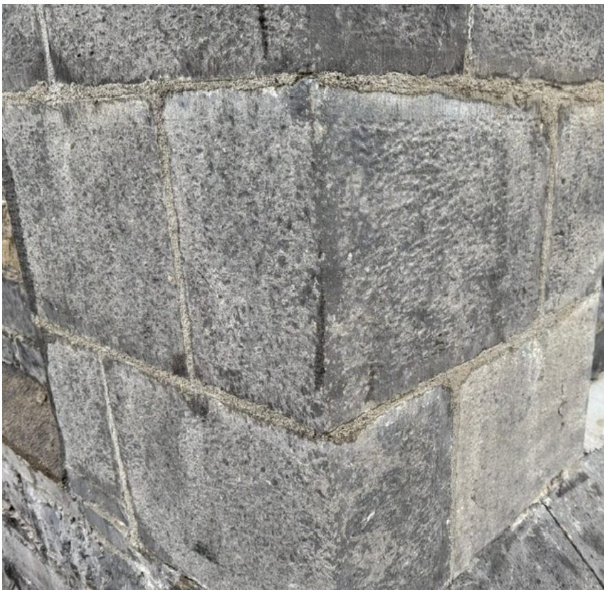
Re-pointed stonework on corner of tower
