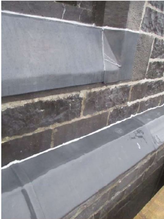
Detail of lead linings to string course and sill under louvred opening of belfry
