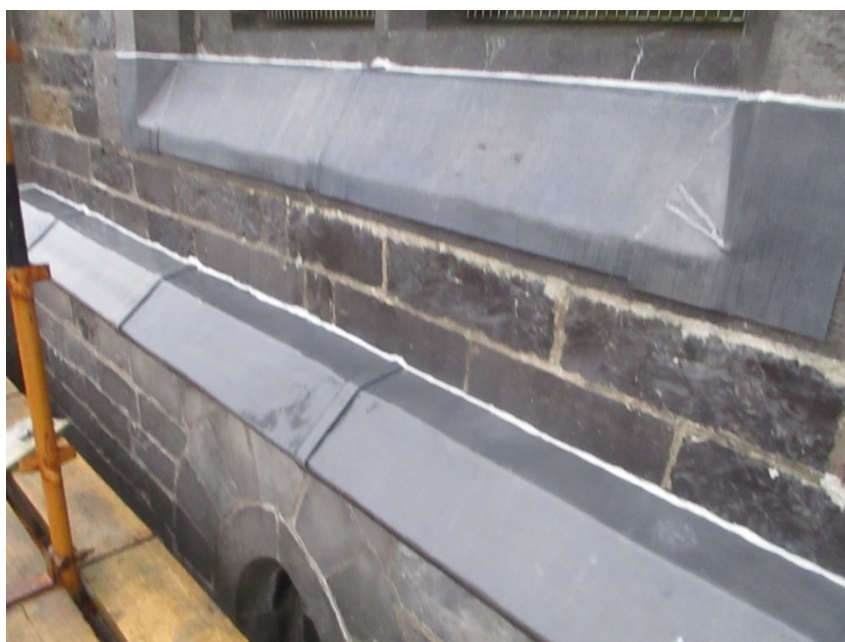
Detail of lead linings to string course and sill under louvred opening to the belfry
