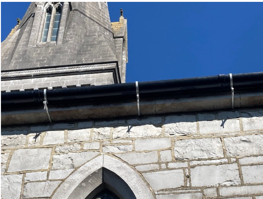
Detail of completed gutter and replacement brackets
