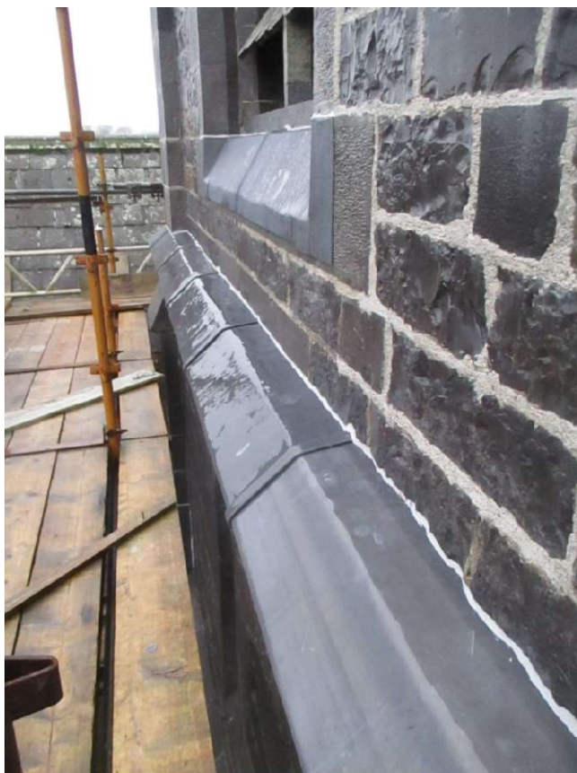
View of completed lead linings to sill and string course on SE face of tower. Some lime mortar pointing of stonework is also pictured to the RHS
