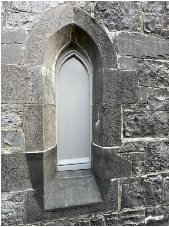
Original door and frame repaired and re-fitted in tower
