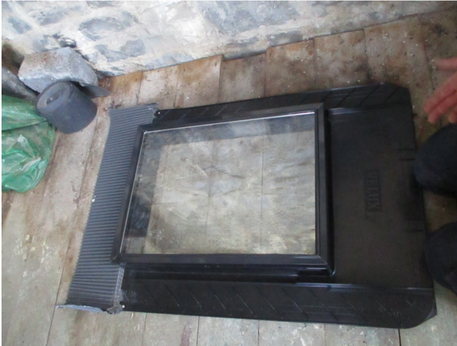
New access hatch being prepared for installation in roof
