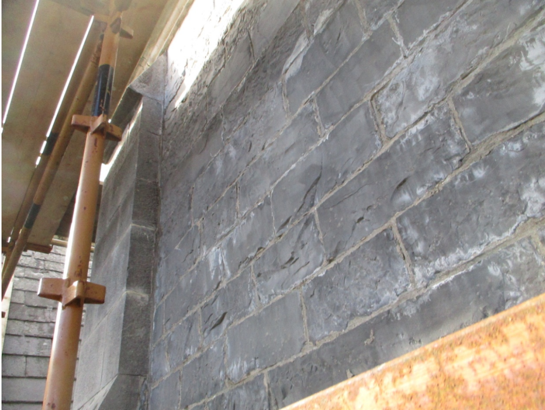
General view of re-pointing of masonry on tower
