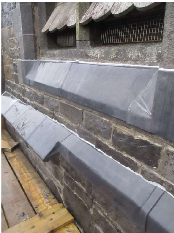
Detail of lead linings to string course and sill under louvred opening of belfry on the SW face of the tower.
