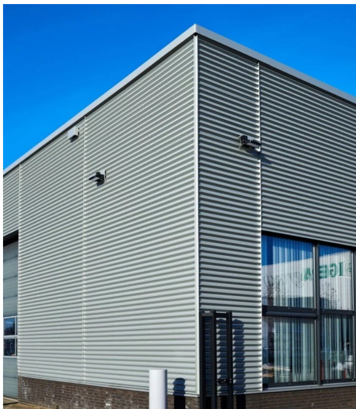
ISIS Custom-made - Renovation Tiel Hairexcel 6906 (9006)
