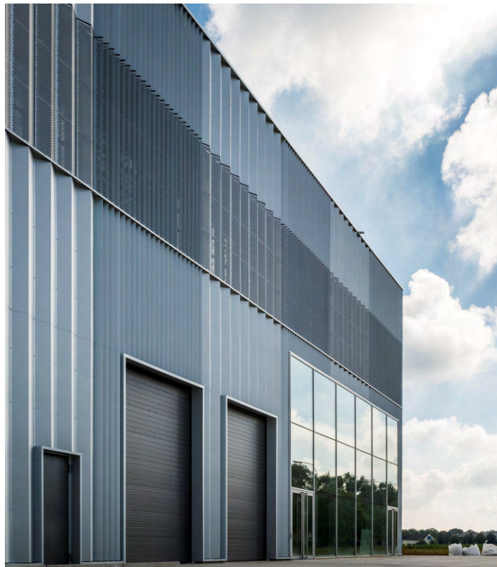
Deca Packaging - Herentals Architect: 2DVW architecten bvba
