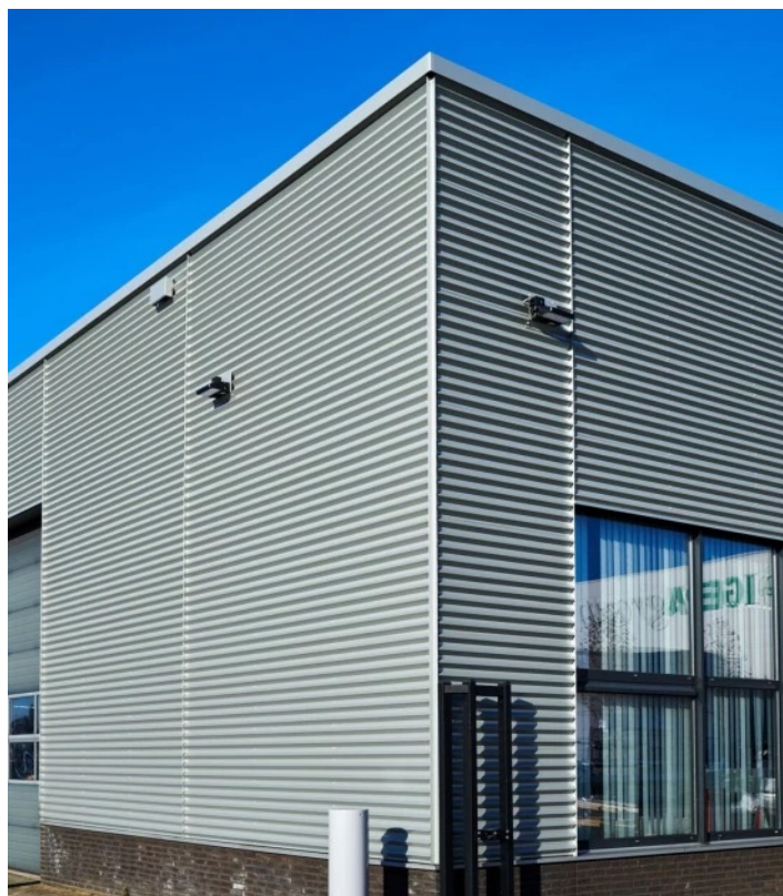
ISIS Custom-made - Renovation Tiel Hairexcel 6906 (9006)
