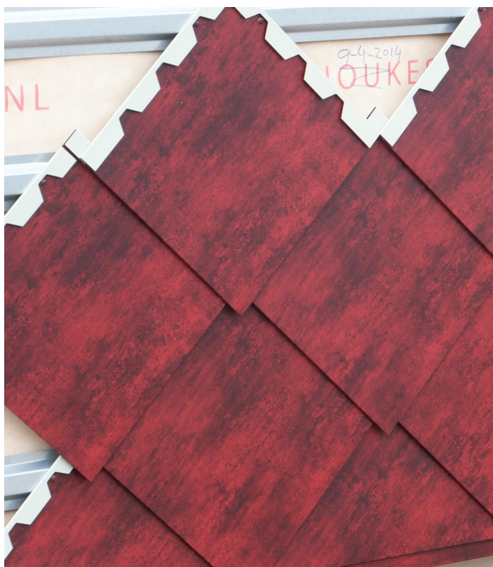
Detail Korfvis Urk - Flat Lock system Intense Bronze 1829
