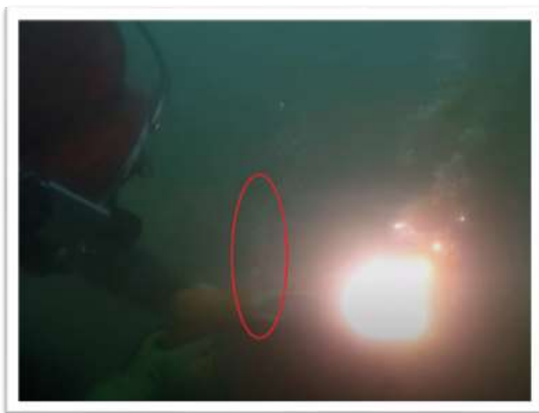
Fig. n° 58: Cutting hot = H_2 formation at the rear side of the rod (78).
