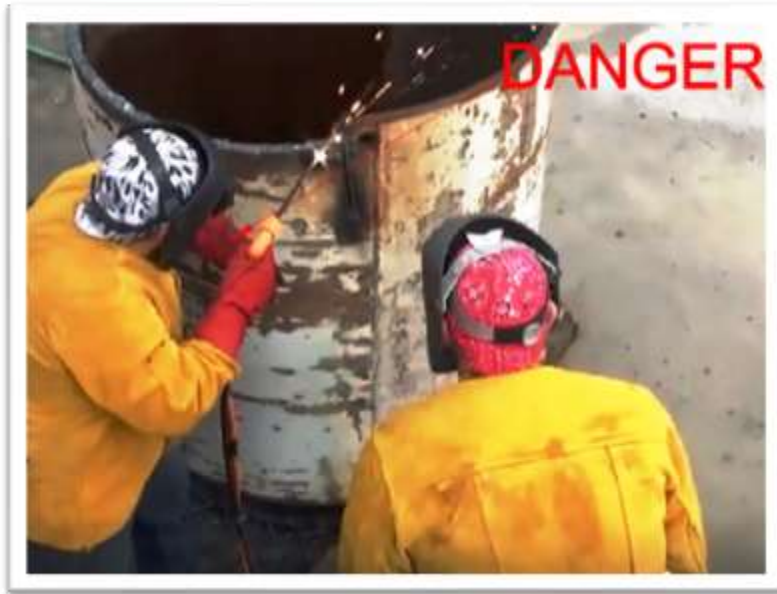
Fig. n° 52: Avoid being in contact with the structure (72)
