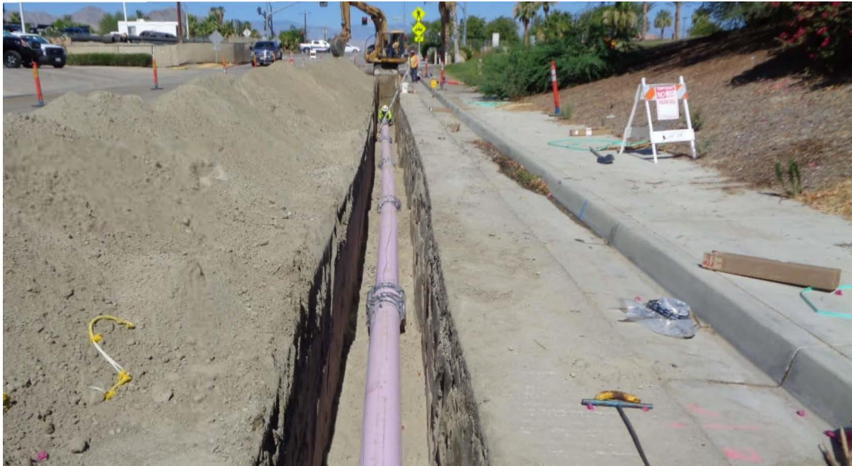
Figure 4 Typical Non-Potable Water Pipeline Trenching Work Site
