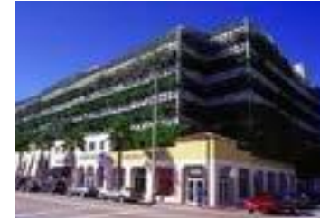
MIAMI PARKING GARAGE
