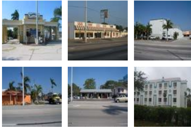
Building condition varies greatly along the corridor
