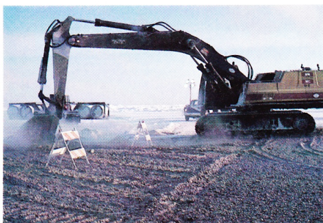
Backhoes are used to remove the individual ice blocks, some of which weigh more than 8,000 pounds, from the checkerboard.
