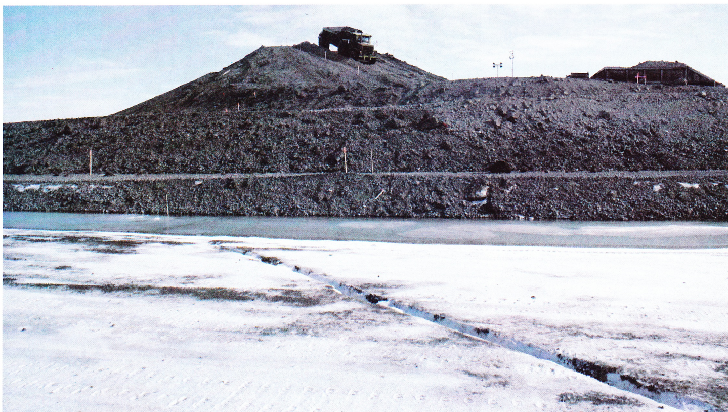
A mountain of gravel — 20,000 truck loads of it — rises from the sea as construction workers complete the construction of Seal Island.
