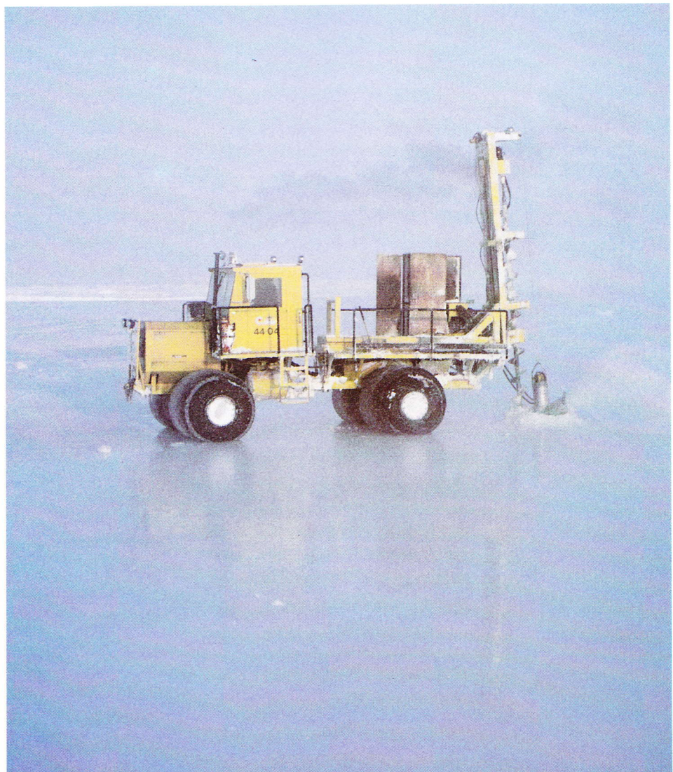
Water is pumped onto the ice surface where it freezes, building up the road thickness.
