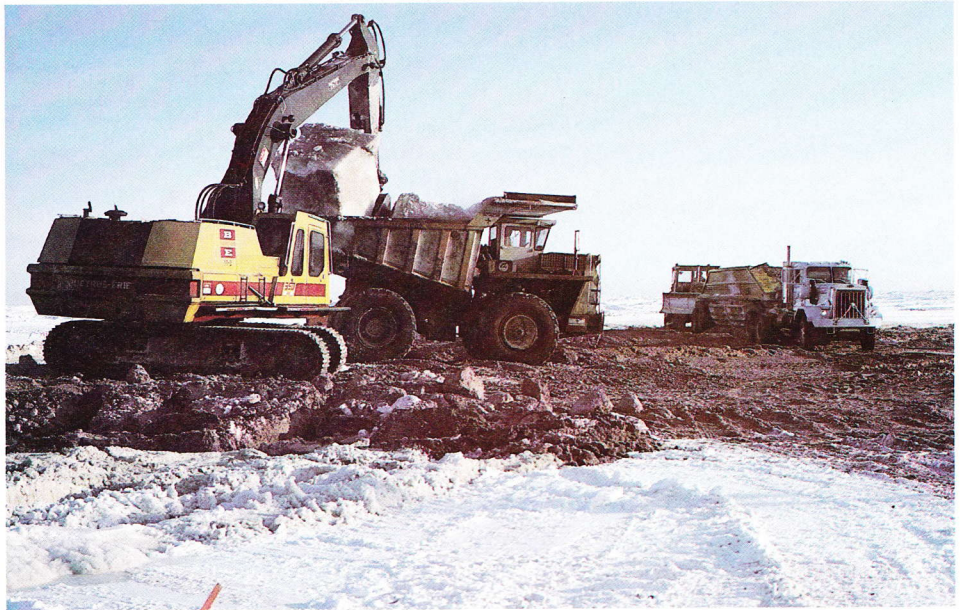
The ice blocks are loaded into gravel trucks and then are hauled off to a dumping site.
