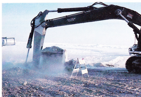
Backhoes are used to remove the individual ice blocks, some of which weigh more than 8,000 pounds, from the checkerboard.
