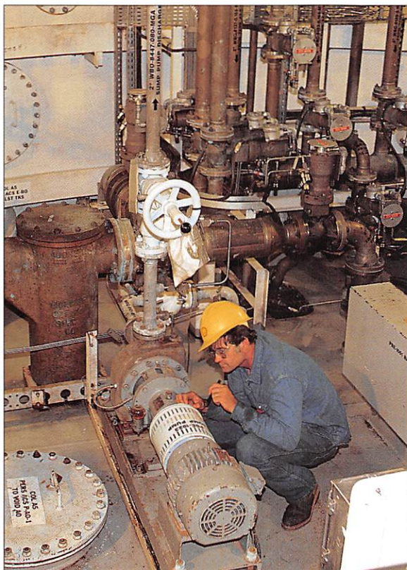
Blue-Yellow team member Joe Whiddon checks a ballast pump on Auger, an innovative tension leg platform.
