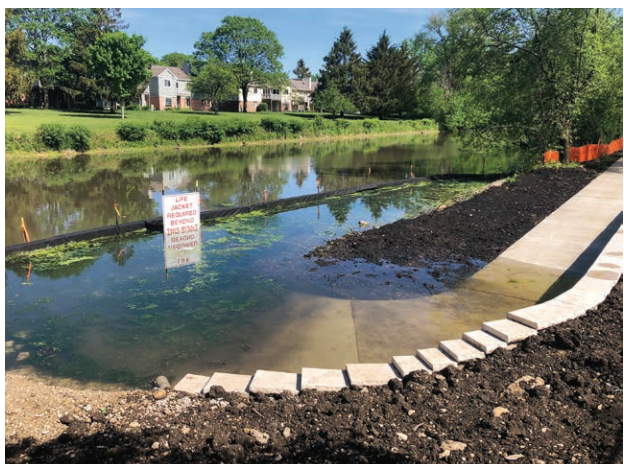
Winfield's new DuPage River canoe launch is under construction.
