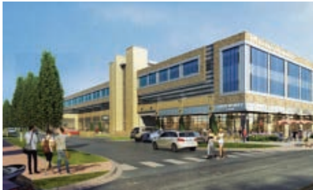
Rendering of new downtown parking deck under construction on the former site of John's Buffet.
