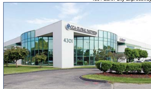
4301 Earth City Expressway
