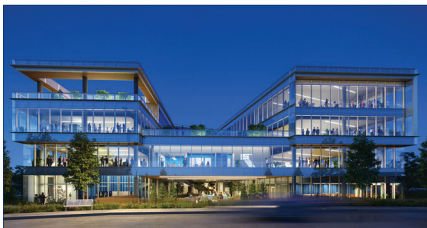
First Bank HQ 11901 Olive Blvd
