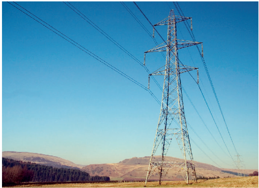
Figure 4.5 Transmission line steel pylon.
