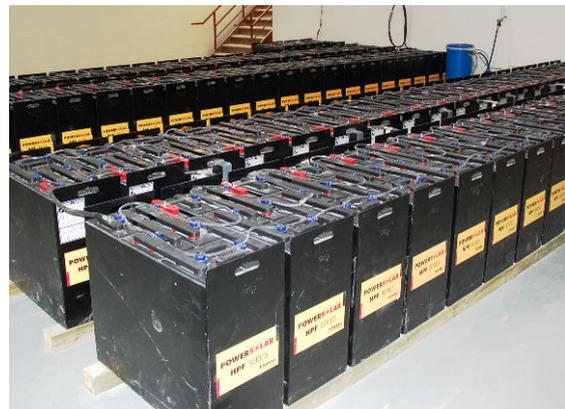
**Figure 2-1.** A battery array providing 60KW at 480VDC as backup for a corporate data center. (Photo by permission of Hybridyne Power Systems, Canada, Inc., and the Hybridyne group of companies. Copyright by Hybridyne, an internationally registered trademark of Hybridyne Power Systems Canada Inc. No right of further reproduction unless specifically granted by Hybridyne.)
