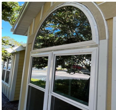
Arched window, with the central and the horizontal aluminum mull bars without the outside clipped snap trim finishing.
