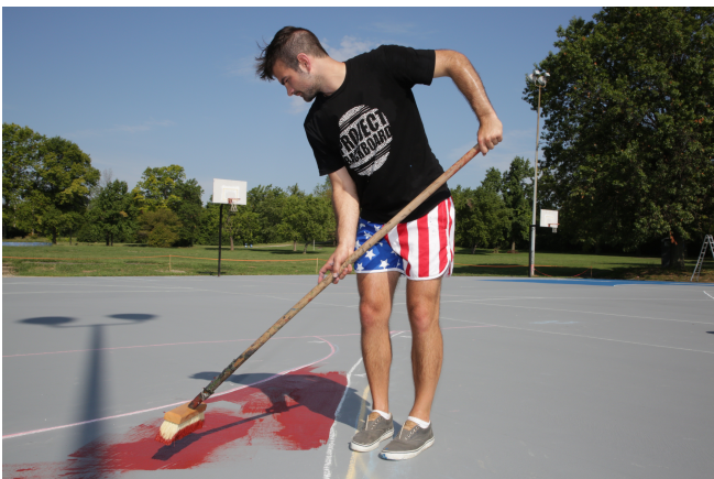
Use roofing brushes for smaller sections
