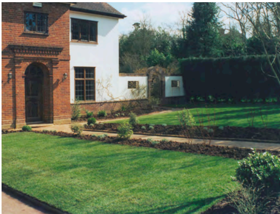
Photo2: View of the property front from the road.
