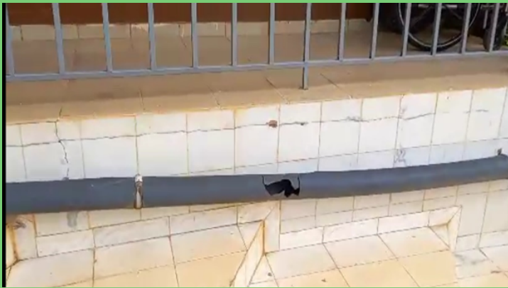
Damaged pipes on ground floor and roof
