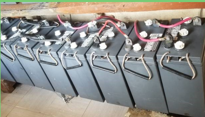
Solar batteries need to be replaced/upgraded
