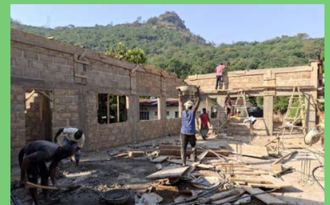
Constructing walls on 2 nd floor
