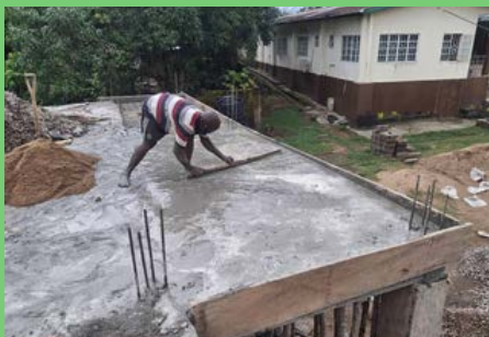
Working on foundation for 2 nd floor
