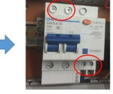
2.Loose four screws of the circuit breaker (in the red circle),
