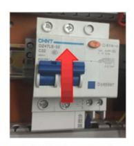
3. Push the breaker upward to remove it.
