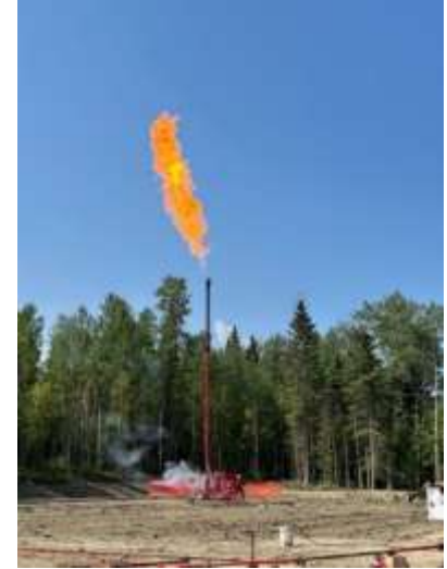
Well production test of HBS in Alberta
