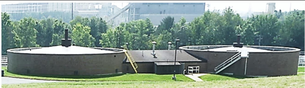
Figure 6.01-10 Anaerobic Digesters
