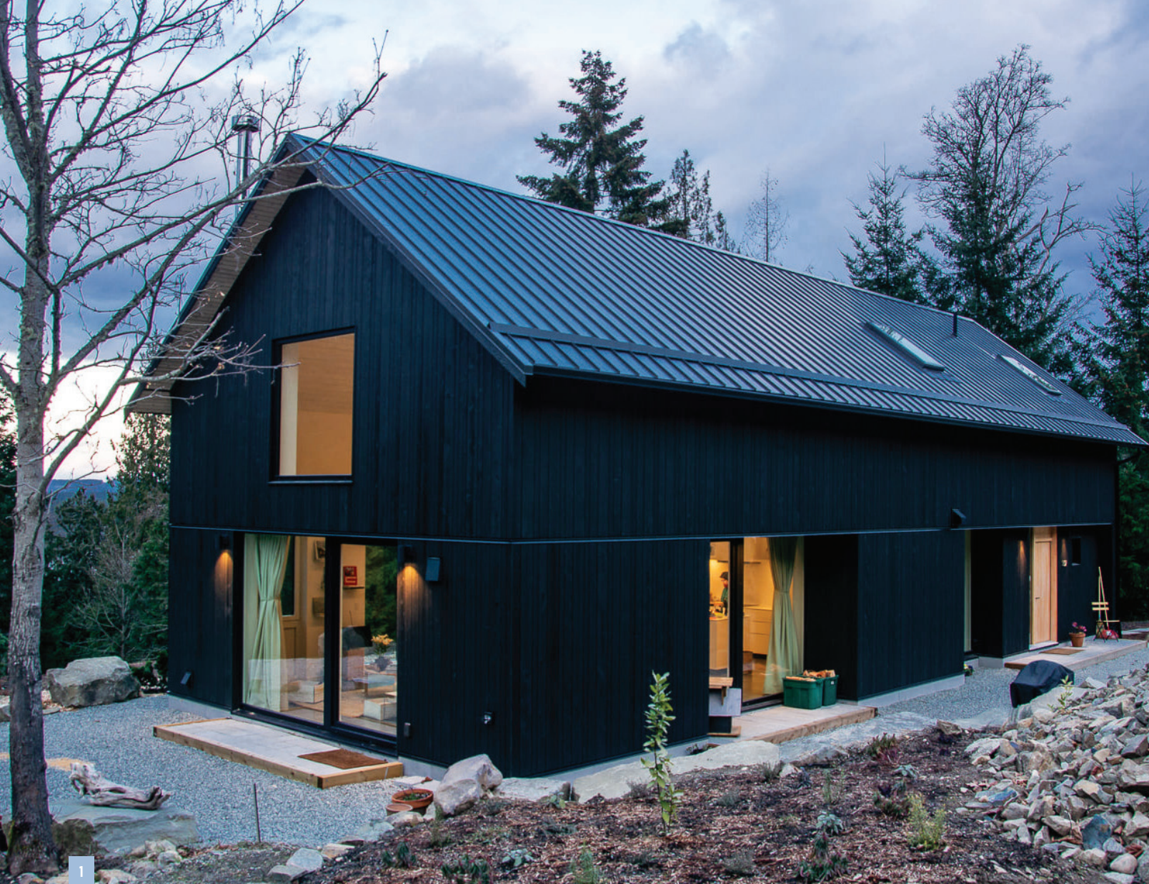
1. Oblique view of the west and south elevations. The vertical western red cedar siding was factory pre-stained.
