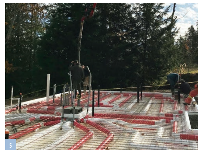
4. The narrow footprint allows plenty of natural light throughout the interior. 5. Installing the in-floor warm air radiant heating system prior to the slab pour. 6. The master bathroom on the second-floor loft where a skylight admits additional natural light.
