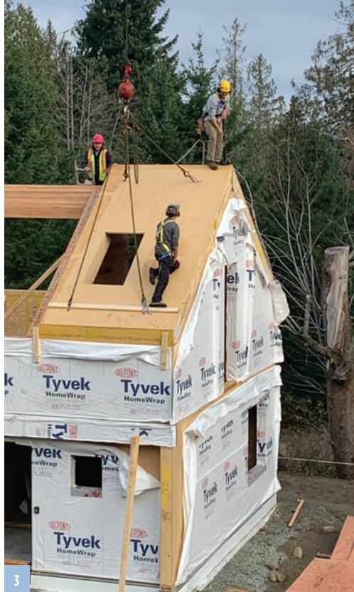
3. The prefabricated wall and roof panels and service wall assemblies provide R values of 32 and 47, respectively.
